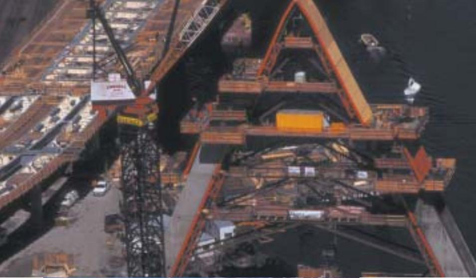
Left: Earlier photo shows Cornell tower crane placing concrete for workers forming inverted-Y tower leg.
