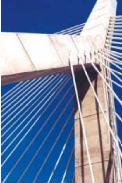
Twelve-inch-thick cable stays are anchored to high-performance grade 70 steel in tower core.
