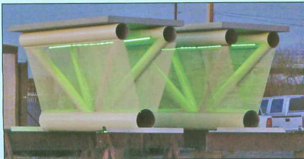
Figure 3: Fabricated full-size mock-up of design with lighting system
