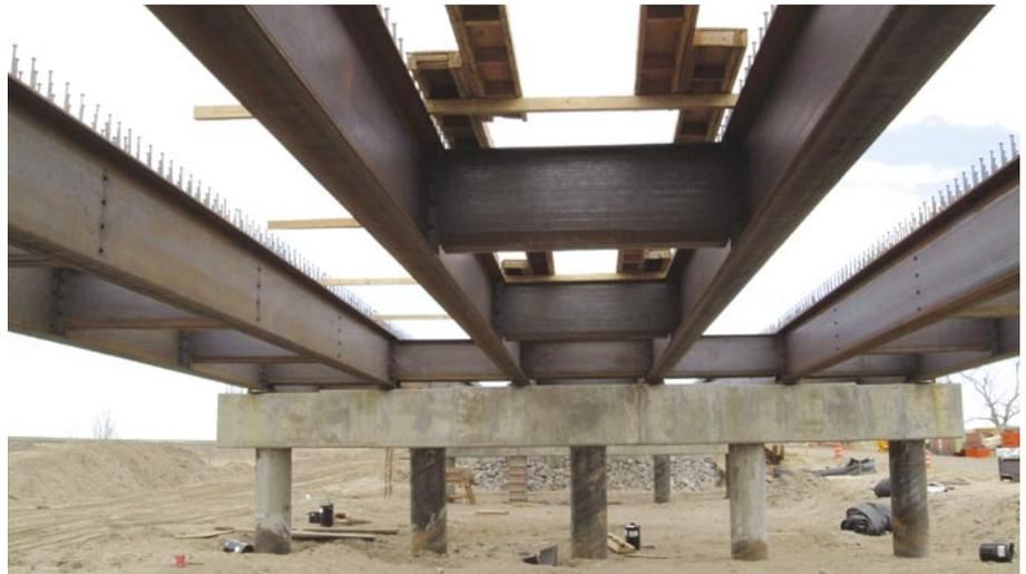
Rollled beam girders and diaphragms form the steel superstructure for the bridge.
