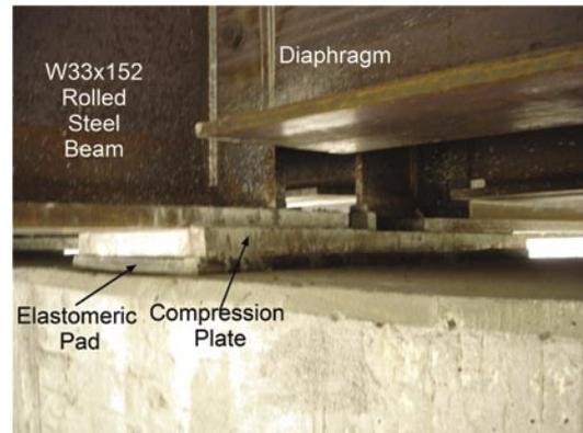
Workers welded the bottom flanges of in-line girders to a compression plate bolted to the pier, creating a continuous connection for live loads.
