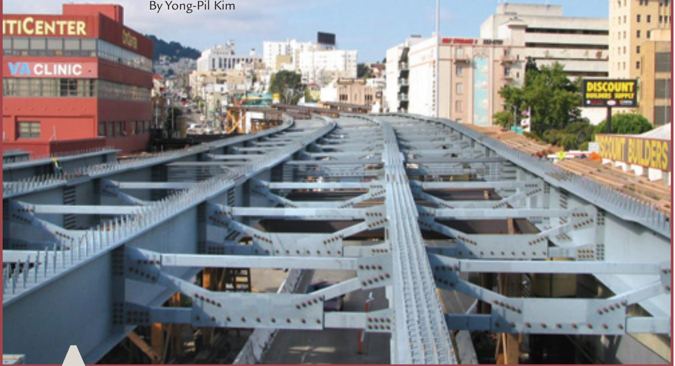
A new Central Viaduct will soon direct traffic into San Francisco from the Bay Bridge in the east and from Highway 101 in the south. The new steel viaduct replaces a previously retrofitted viaduct whose structural integrity came into question after the 7.1-magnitude Loma Prieta earthquake in 1989. After the earthquake, Caltrans removed the upper deck portion of the viaduct in the interest of safety.
