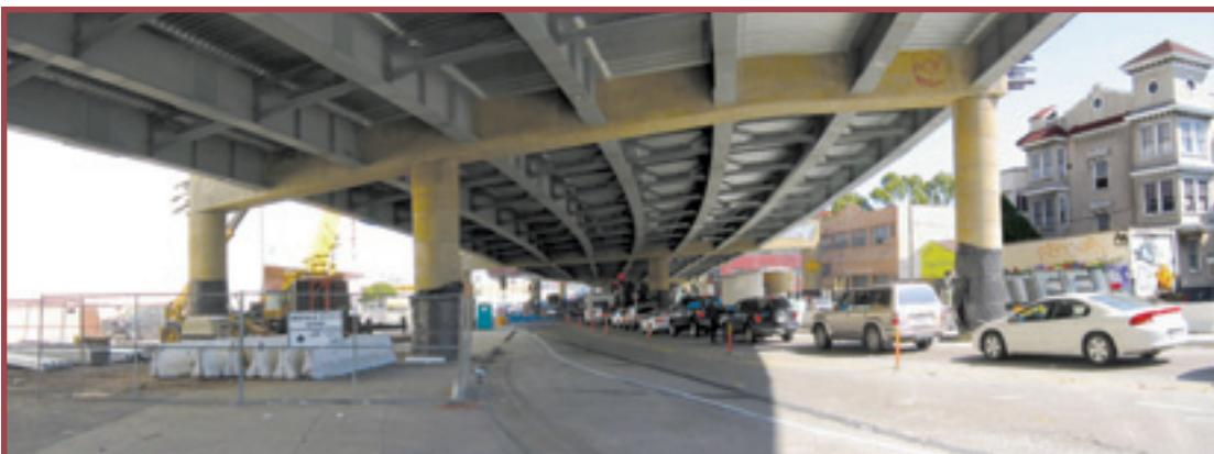
The continuous steel girders are integral with the concrete bent cap to provide vertical clearance near 17 feet at the lowest point.
