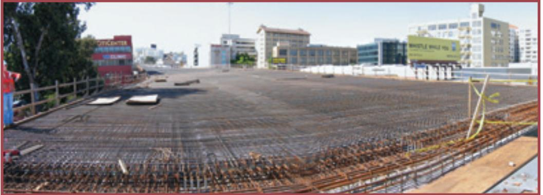
The deck pan varies from about 9.5 inches to 10 inches thick, depending on the girder spacing. The contractor chose stay-in-place metal forms for the deck pour.
